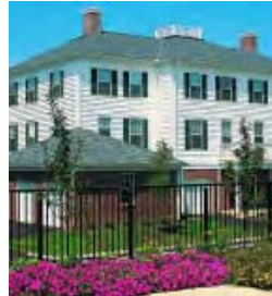
The balcony railing shown on roof top is Series 990 with Superior panel column posts. The railing shown in foreground is Series 900.
